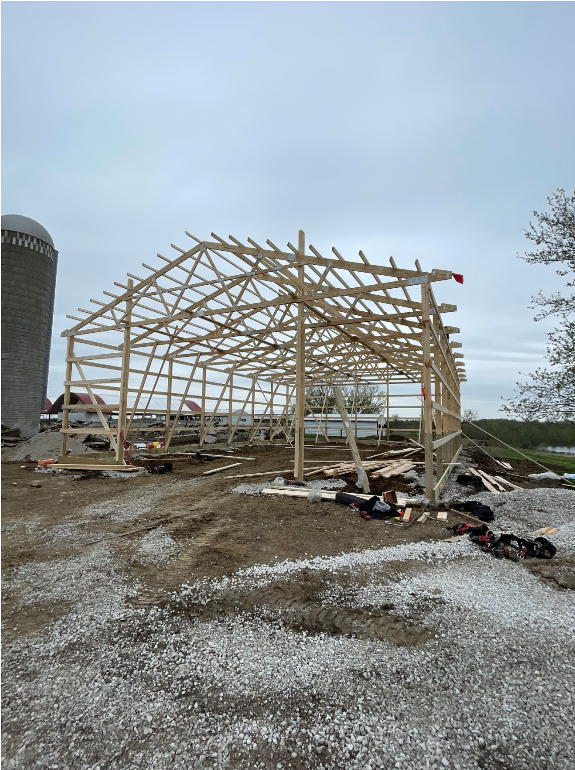
The framework of the building was put up very efficiently.
