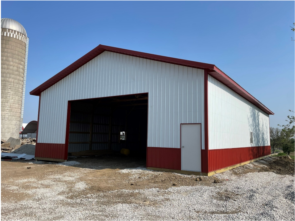
The processing facility is almost complete!
