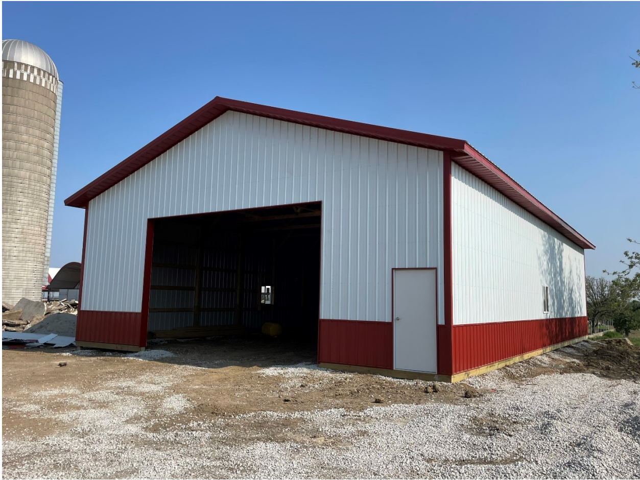
The processing facility is almost complete!
