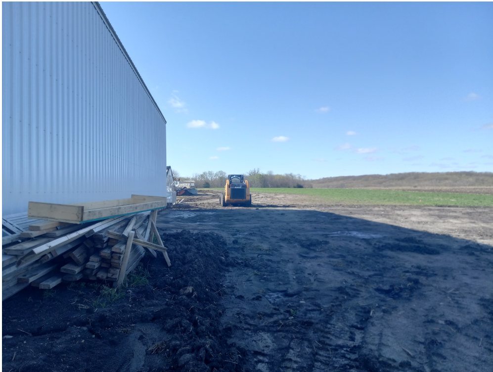
Before the shipping containers could arrive, the land had to be prepared.
