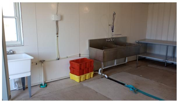
Construction of the pack/wash shed has begun. This large 3 basin sink will allow for easy washing of large quantities of vegetables. A separate hand washing/utility sink is installed to promote goo hygiene/food safety practices for the growing vegetable operation.
