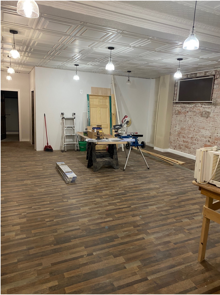
The renovation of the store is in progress and moving forward.
